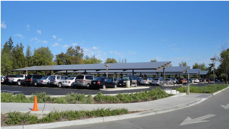
West Valley Community College's parking lot solar system helps provide shade and lower-cost energy for the campus. (Credit: Sunpower/West Valley Community College District)
