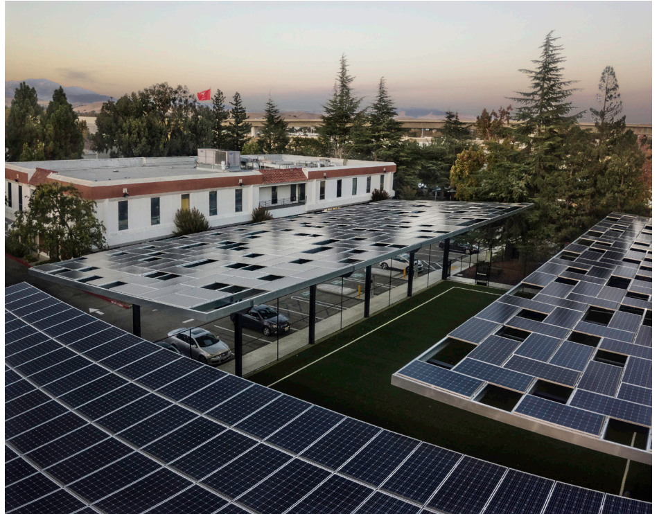
A solar canopy at Fountainhead Montessori school in Dublin, CA. (Credit: Solar Technologies)
