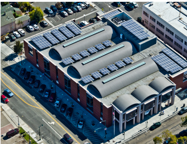
Solar installation at the Alameda Public Library. (Credit: Sun Light and Power)
