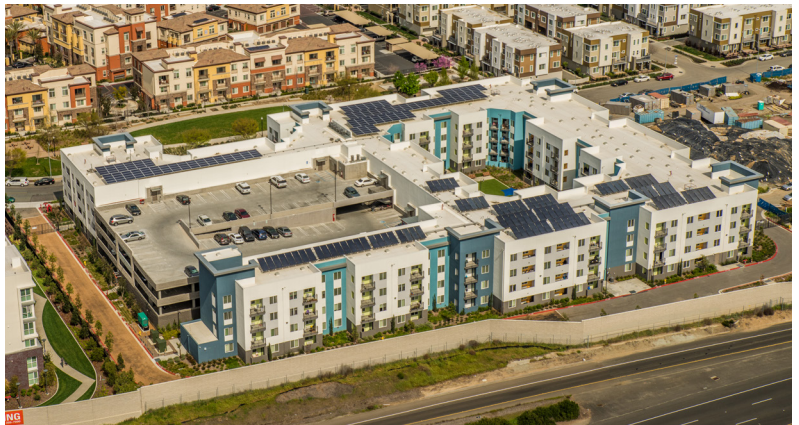
A solar electric and solar hot water system on a low-income housing complex in San Jose, CA. (Credit: Sun Light and Power)
