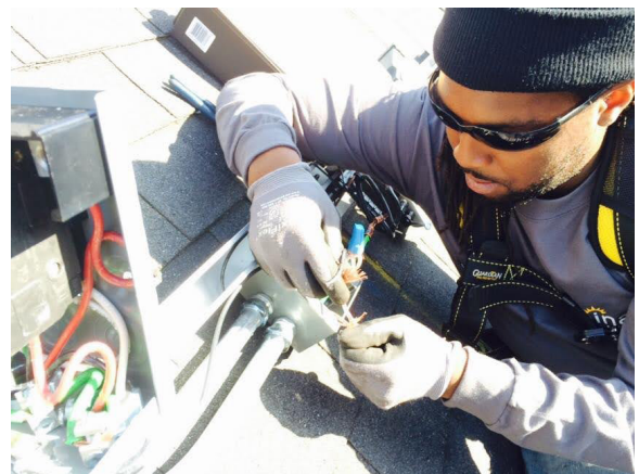
A Luminalt crew member completing an installation. (Credit: Luminalt)
