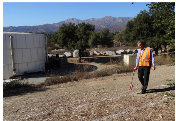
Caption: Bert J. Rapp, General Manager of Ventura River Water District, marks off the area where batteries are to be installed later this year. (Credit: Ventura River Water District)
